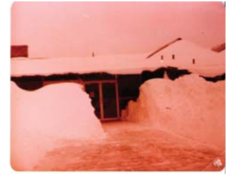
1978 Airport Terminal Baggage Claim
